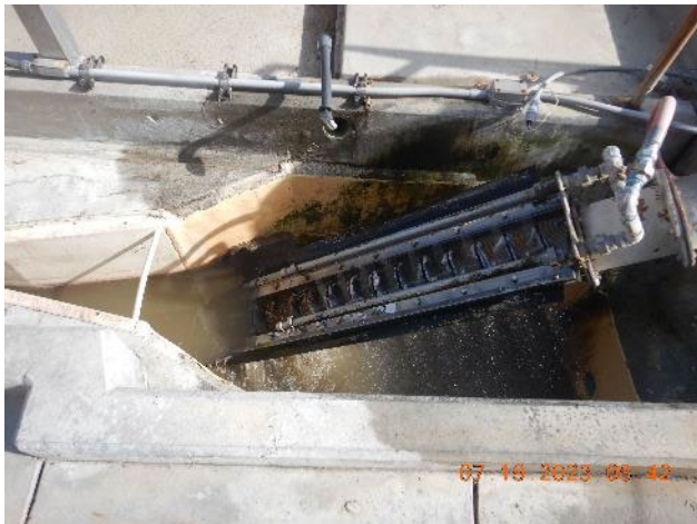
Photos 2 and 3. In channel Auger Monster grinder, screener, and compactor.
