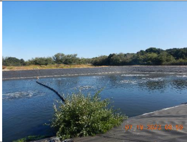
Photo 5. Lined Pond 1. Aerated section.
