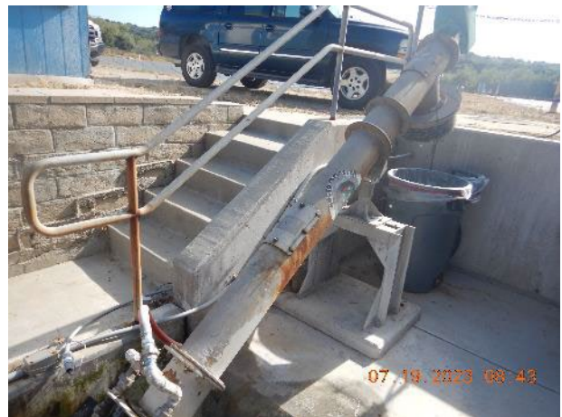
Photos 2 and 3. In channel Auger Monster grinder, screener, and compactor.
