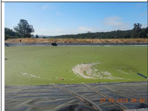
Photo 8. Algae in lined Pond 2.
